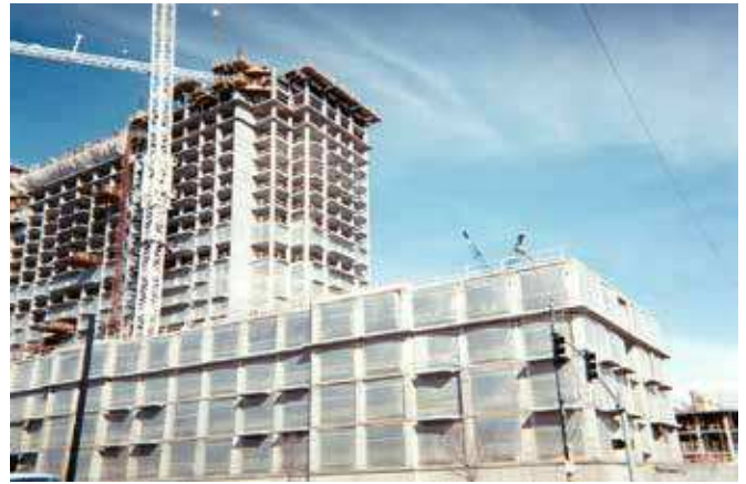
Building Abatement Enclosure
